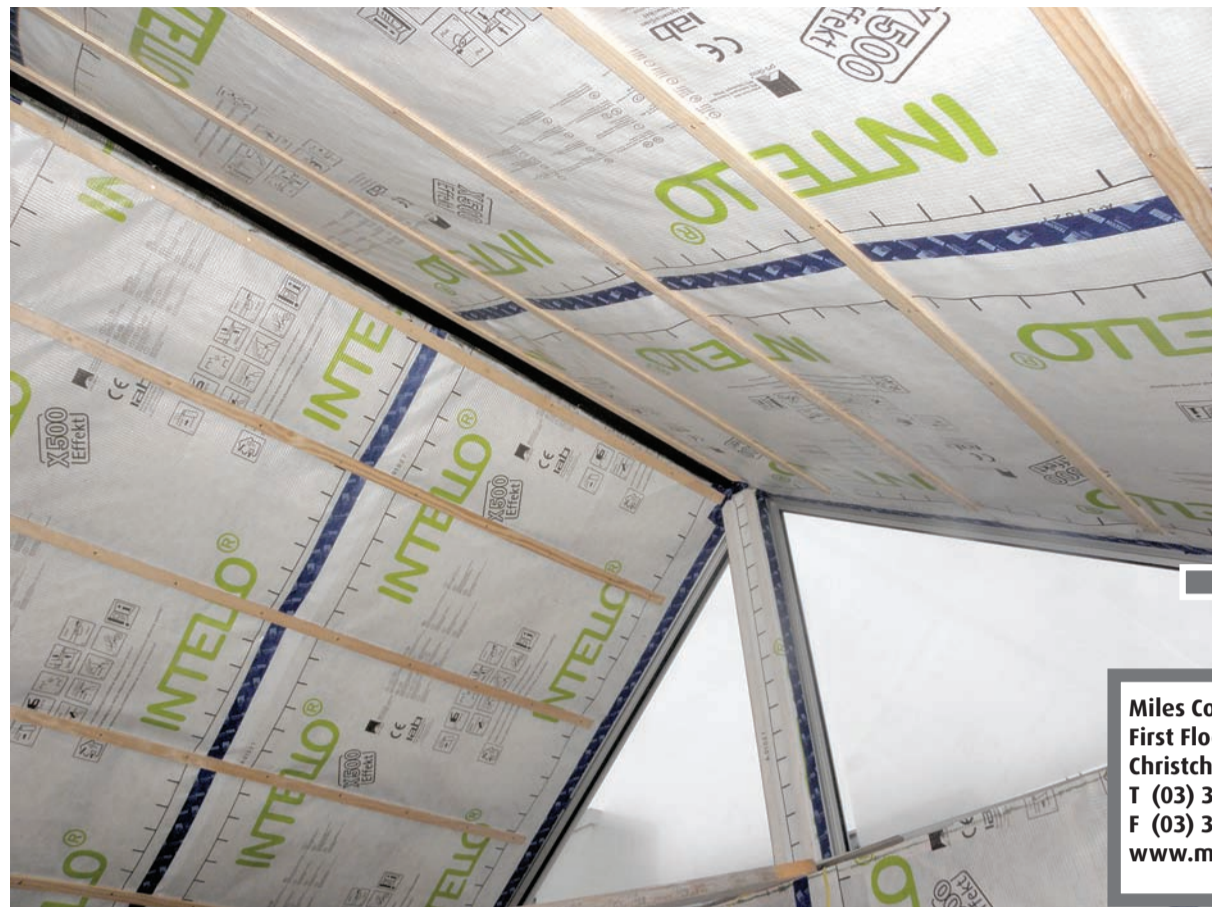
LEFT: The unique Intello Plus building wrap used by Miles Construction
